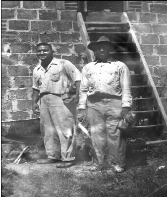
Herbert (left) and Clarence Brown, a bricklayer, began building a home at 5901 Clay St., N.E., in Washington, D.C., in 1947. Herbert was the first Black deaf person to build his own home in D.C.
