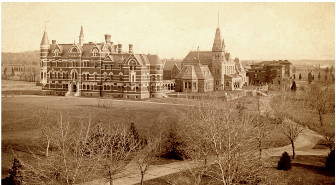
This western view of Kendall Green shows College Hall (left, completed 1877), Chapel Hall (center, completed 1871), and "old" Fowler Hall (right, completed 1859). Both Chapel Hall and the west wing of College Hall were designed by Frederick C. Withers. The east wing of College Hall was originally called the "Friedrich building" (for its architect) and "the college building." Photograph circa 1888.
